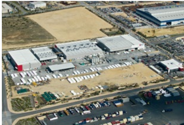
ABOVE: Located in the Australian Marine Complex, the southern hemisphere's premier integrated marine industrial facility
